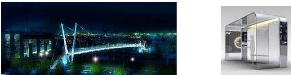
Figure 21 –Footbridge in Paris (credit CSTB) and bus stop with interactive service (MIT project)
